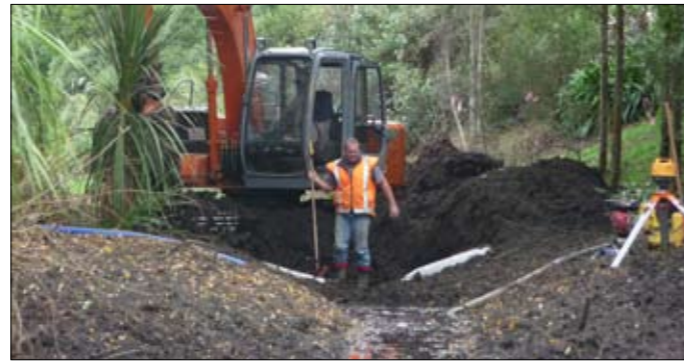
Dormer Construction creating the swale, April 2009.
