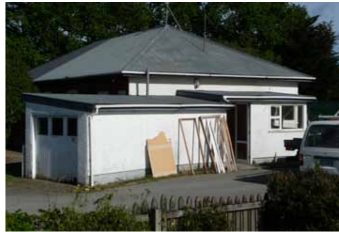
Travis education centre before renovation.
