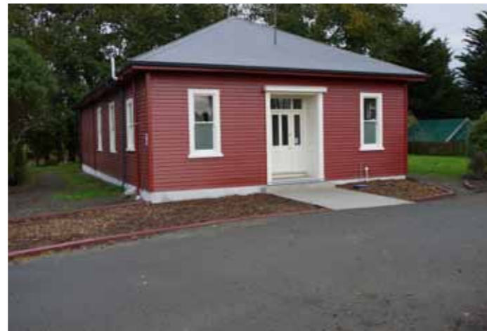
Travis education centre following renovation.
