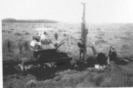
Pile driving near Anne Flanagan Dell.
